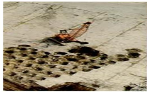
Fig.1 Dynamic Compaction
