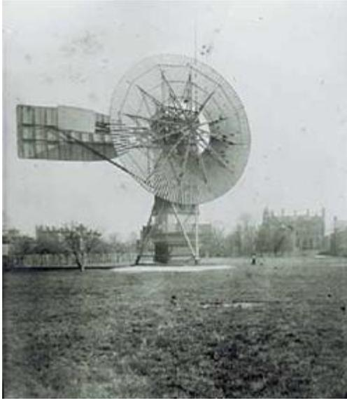
Figure 2. Charles turbine (1887, Cleveland, Ohio), the world's *automatically* first *operating* wind turbine for electricity generation.
